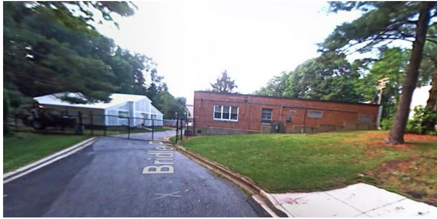
Bowie Water Plant
