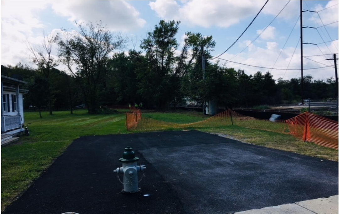
BEFORE: Southeast view from 11 TH Street
