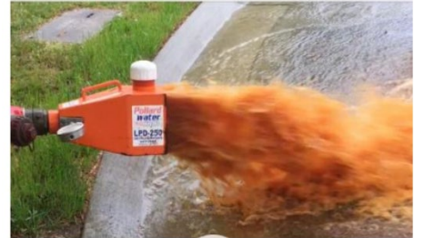
Hydrant Flushing, City of Bowie
