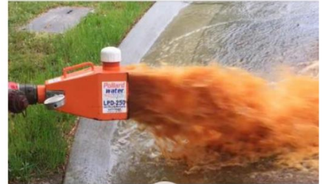
Hydrant Flushing, City of Bowie
