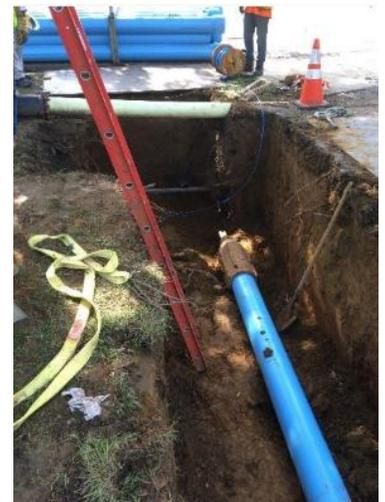
**Heather Hills:** After completion of a hydraulic analysis, 0.4 miles of piping has been identified to be replaced along Hillman Place and a large section of Holiday Lane. This project will include some ‘open cut’ work (pipe expose by digging), and some pipe bursting as described above.
